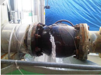
Removal of insulating blanket in summer, failure to reinstall for winter.
