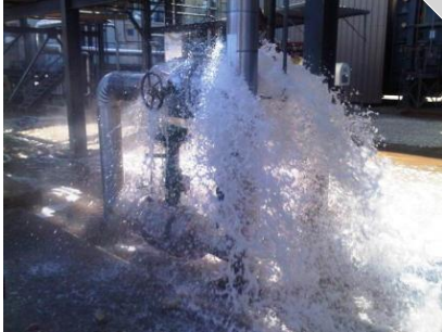
Removal of insulating blanket in summer, failure to reinstall for winter.
